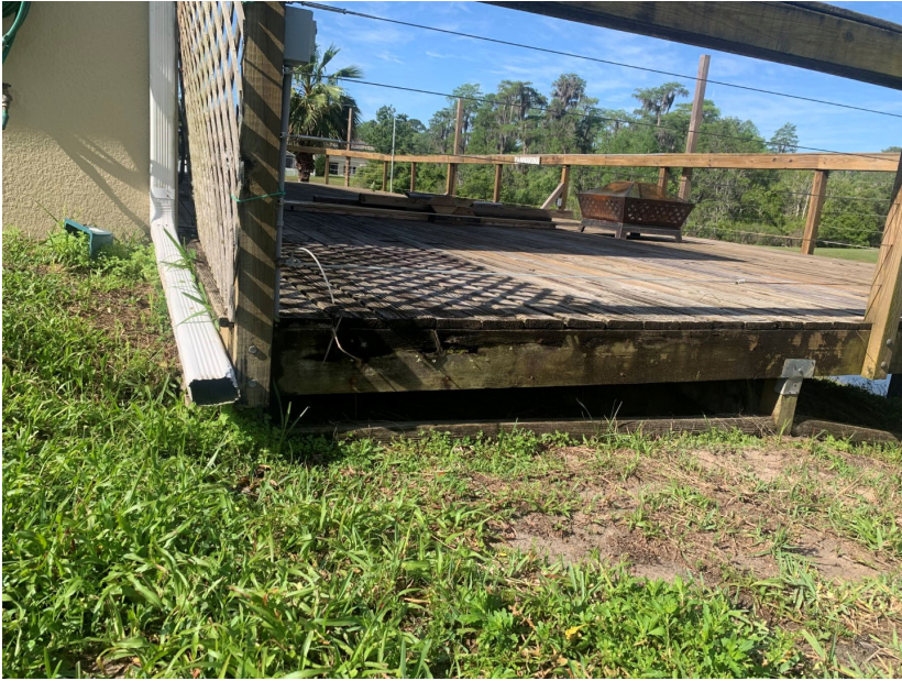
Channelized erosion present beneath deck.
