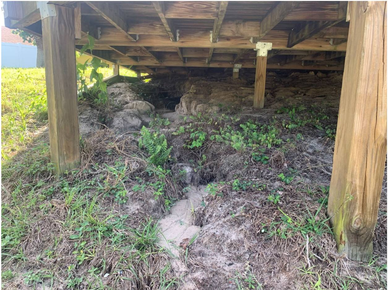
Channelized erosion present beneath deck.
